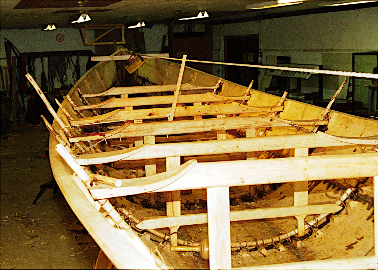
Fig. 6: The Frame Assemblies Mounted in the Boat, Looking aft.
